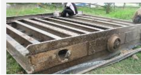
Refurbishment of old water gate at site
