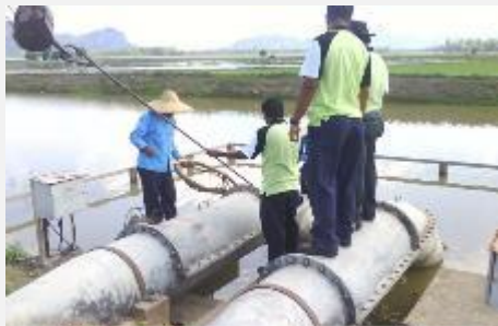
Installation work of ESP at site
