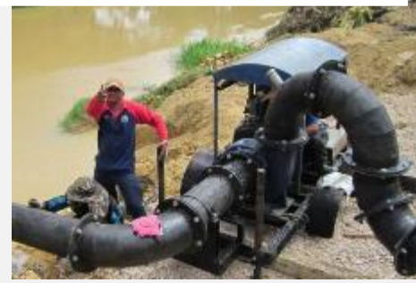
Instalation of 10" pump with engine at site
